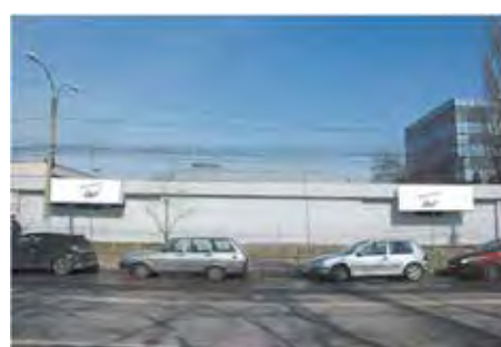
BANNER DISPLAY ON ROMEXPO HEADQUARTER FACADE
